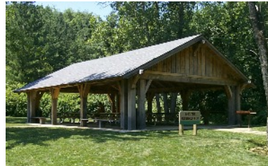
Plum Creek Park South 80-person occupancy
