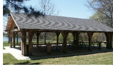
Hubbard Valley Park 80-person occupancy
