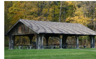
River Styx Park 80-person occupancy
