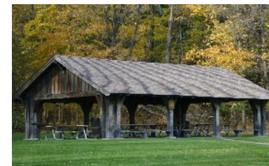
River Styx Park 80-person occupancy
