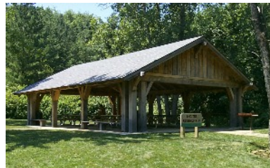
Plum Creek Park South 80-person occupancy
