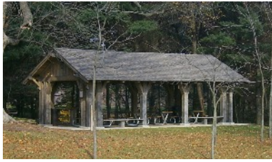
Allardale 32-person occupancy
