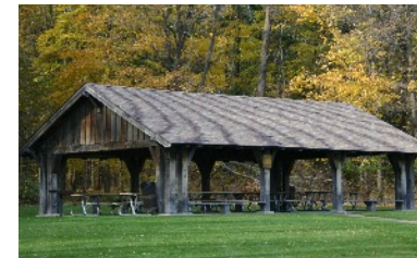
River Styx Park 80-person occupancy
