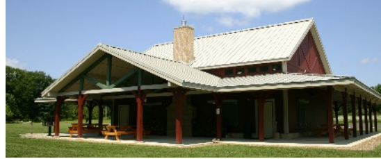
Hidden Hollow Camp 75-person occupancy
